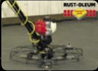
Arlington, TN, USA Walker Composites, Inc. Rust-Oleum FlorClad
